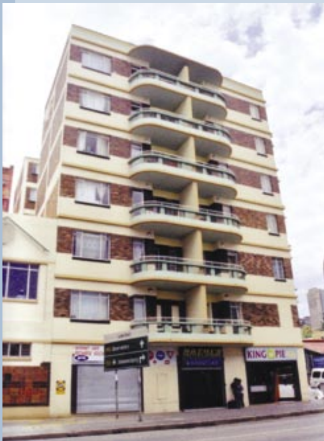
Commercial units take up the ground floor of the New Europa House
