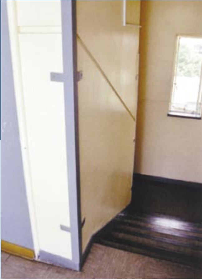
Metal angle fixed to corners reduce common wear and tear
